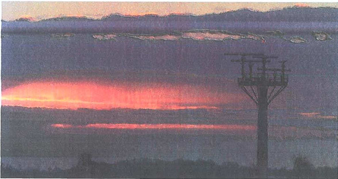
Figure 4-1 Radar test tower at Terma in Lystrup, Denmark
